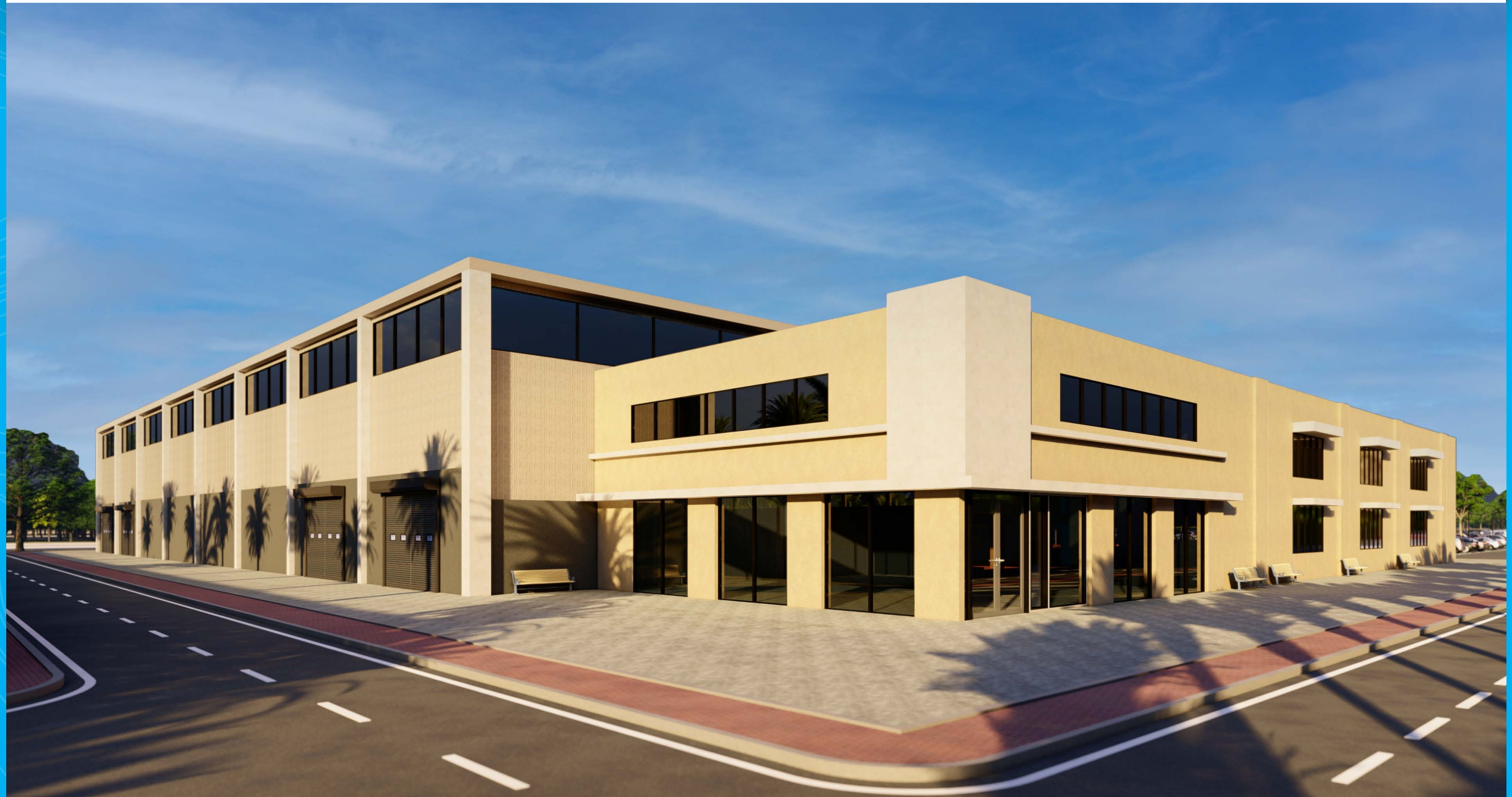
Bayou Phoenix – Back of House
